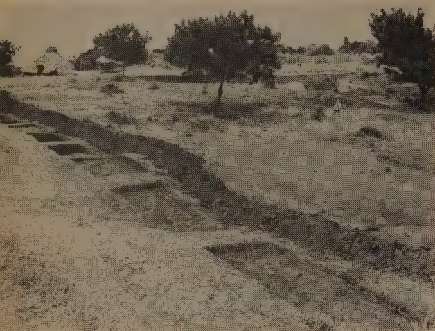
Earthwork basins (called "bunds"). The depressions and mounds break the velocity of run-off water, and trap and retain both water and the soil it carries.
